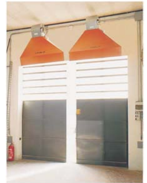
Typical installation of air barriers at malaguti moto in san lazzaro di savena, italy.
