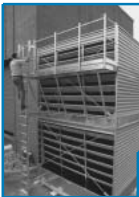
External platform at louver face
