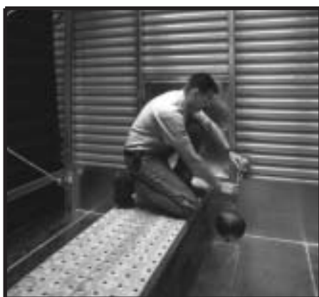
Cold Water Basin Inspection Figure 3
