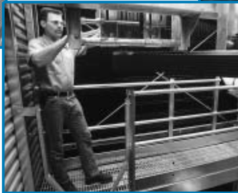
Internal ladder and service platform
